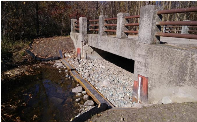
New sheet pile weir structure on upstream (lake side) of bridge
