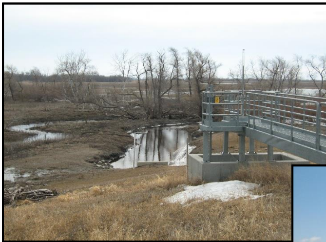
Example of a “Dry” Impoundment. Stored flood water is released as soon as downstream channel conditions are acceptable to pass flows.
