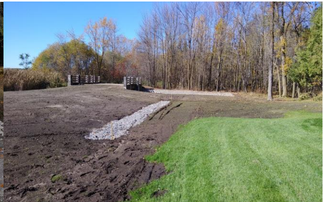
Final grading of approach to bridge. All disturbed areas were seeded and mulched
