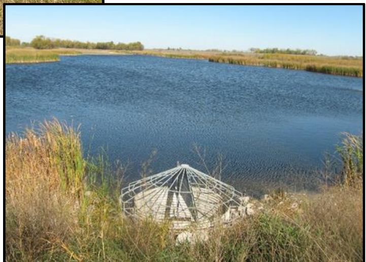
Odney / Flaot Dam located in Onstad Township, Polk County
