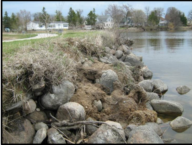
Pre – construction Levee
